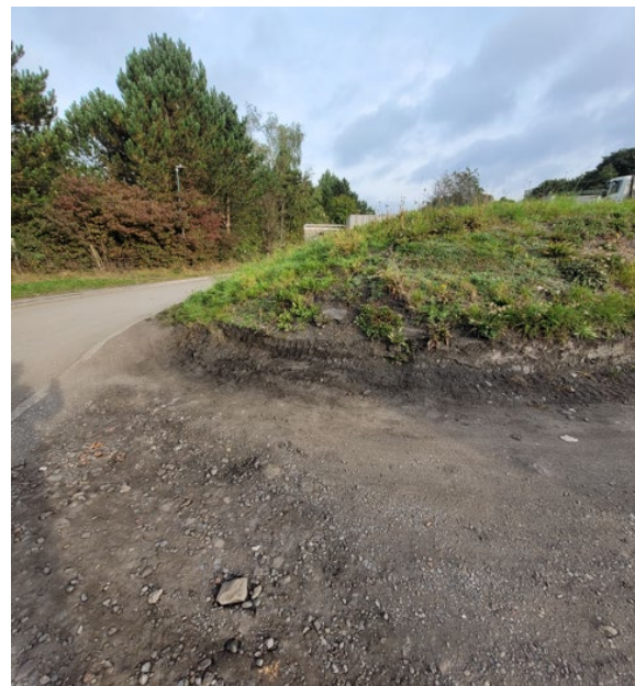
Fig's 13 & 14 (below, L-R) Access track leading up towards the approved site. Visibility splay coming back down the track to turn right onto the highway. Grass mount and garage impede the visibility splay.
