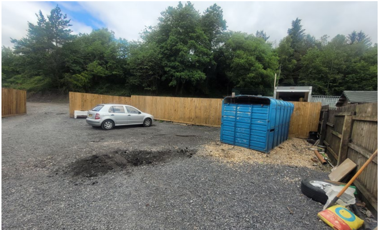
Fig 6: boundary fence erected. Gap in the fence shows an access leading to the land to the north (outside the application site).
