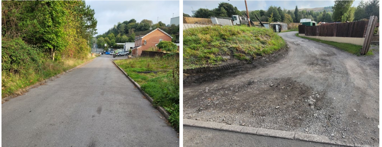
Fig's 11 & 12 (above, L-R) Access road looking northwards and access track leading from the highway in an easterly direction
